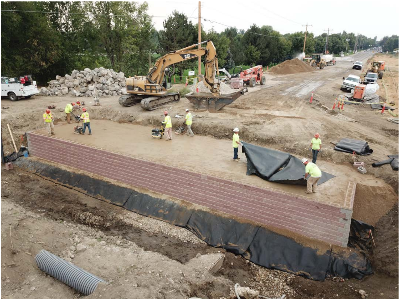
Eagle Rd Bridge 1029
