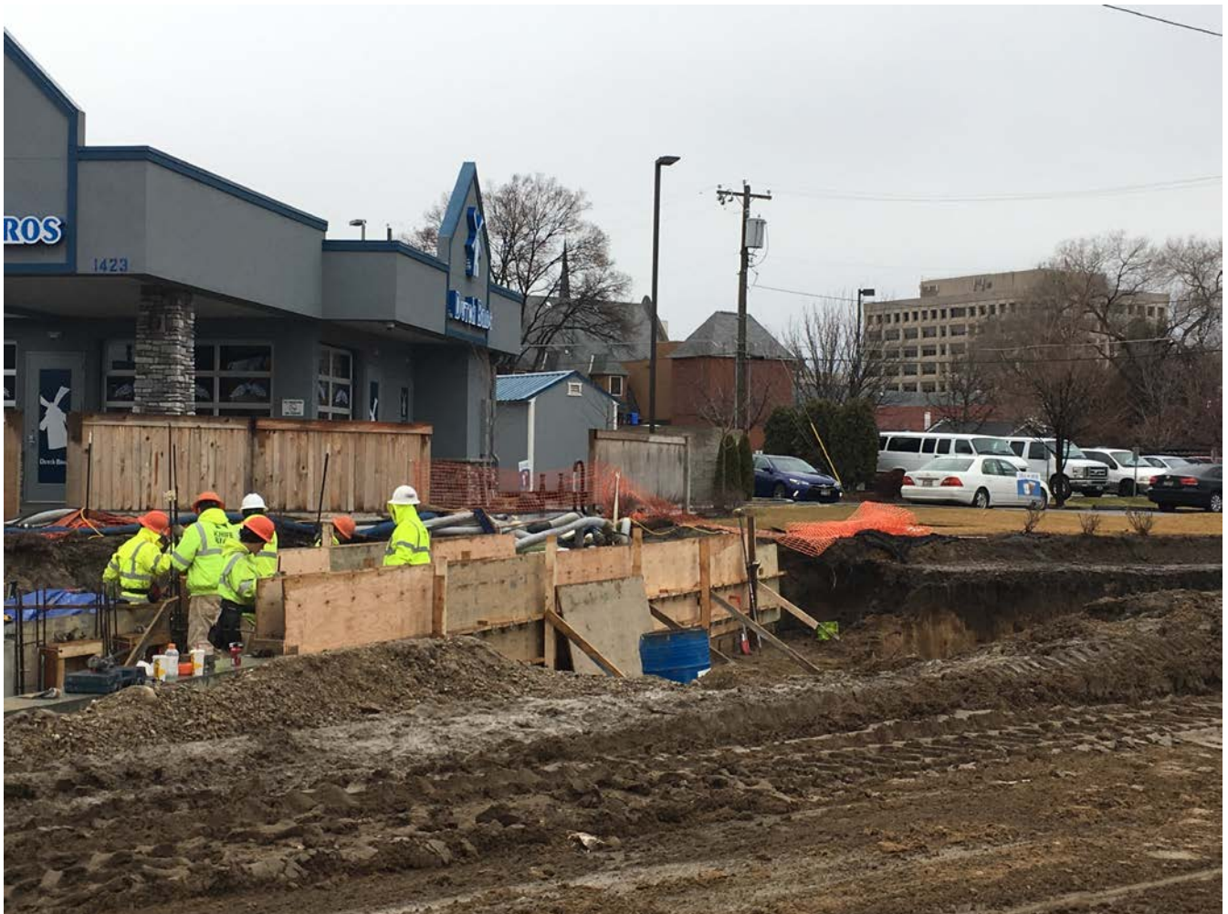
State Street Bridge #1486 at 15 th Street
