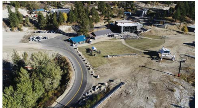
Bogus Basin Rd Maintenance Project
