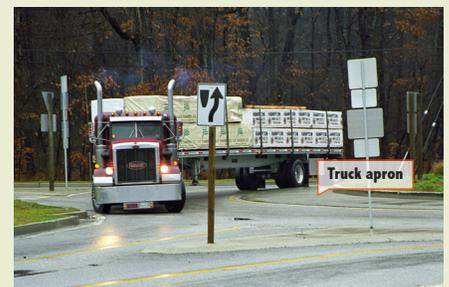
The back wheels of the longer vehicle can ride up on the apron so the trailer can complete the turn; The raised lip of the concrete apron discourages use by smaller vehicles.
