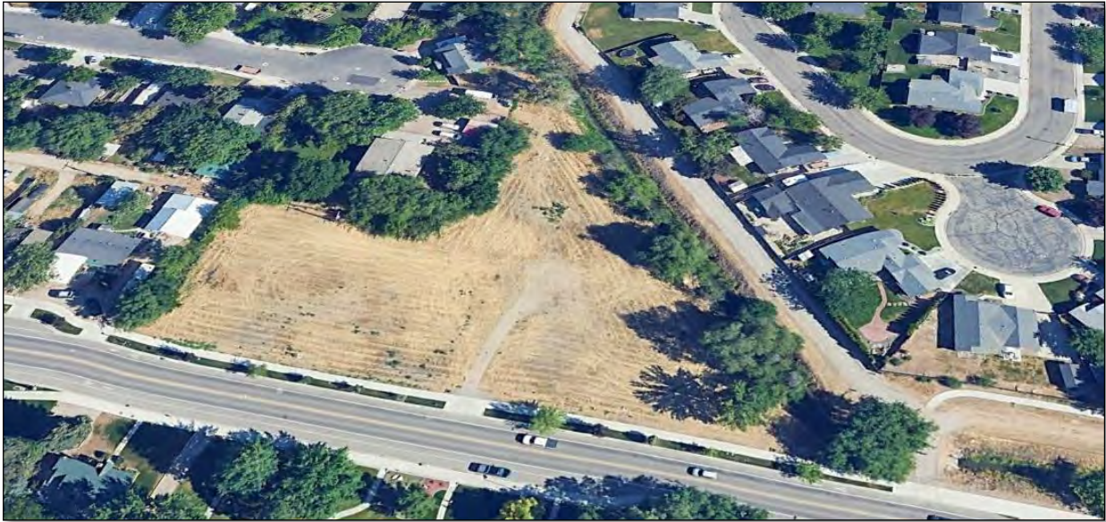
Photo 1: 7/13/2023 - Aerial of basin site (taken facing northwest) prior to construction of the stormwater basin.
