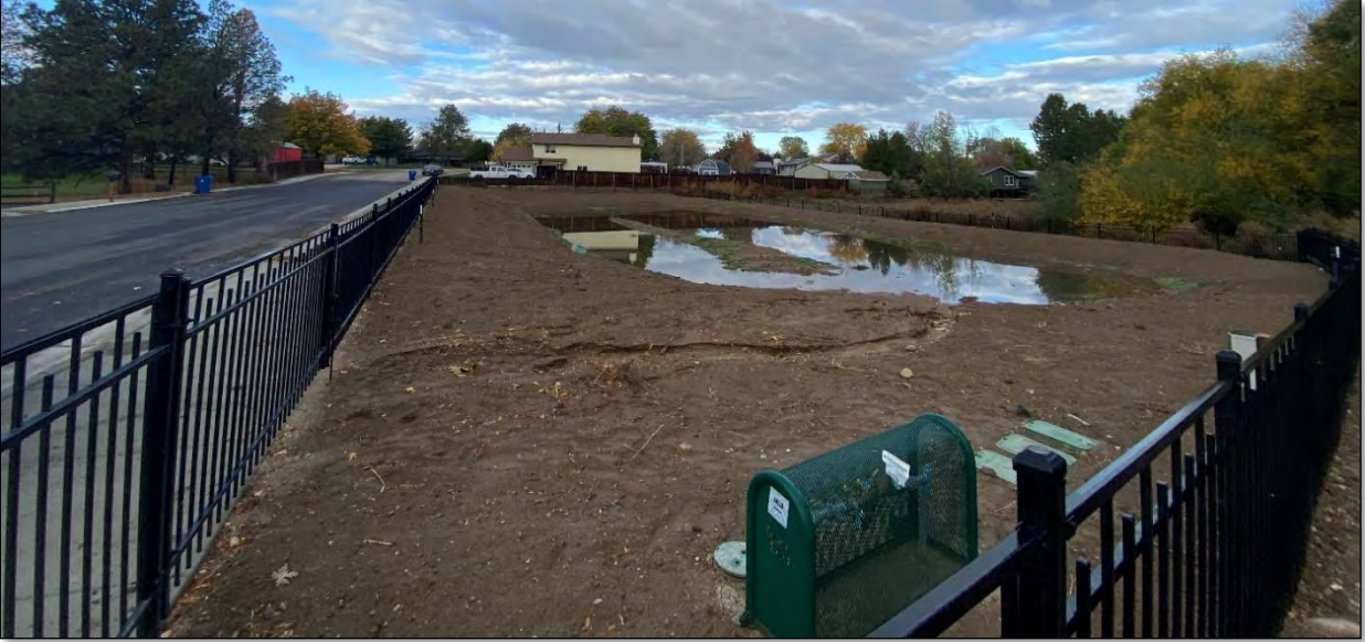
Photo 3: October 2023 – Photo taken facing northwest showing grading, topsoil, and irrigation system complete.
