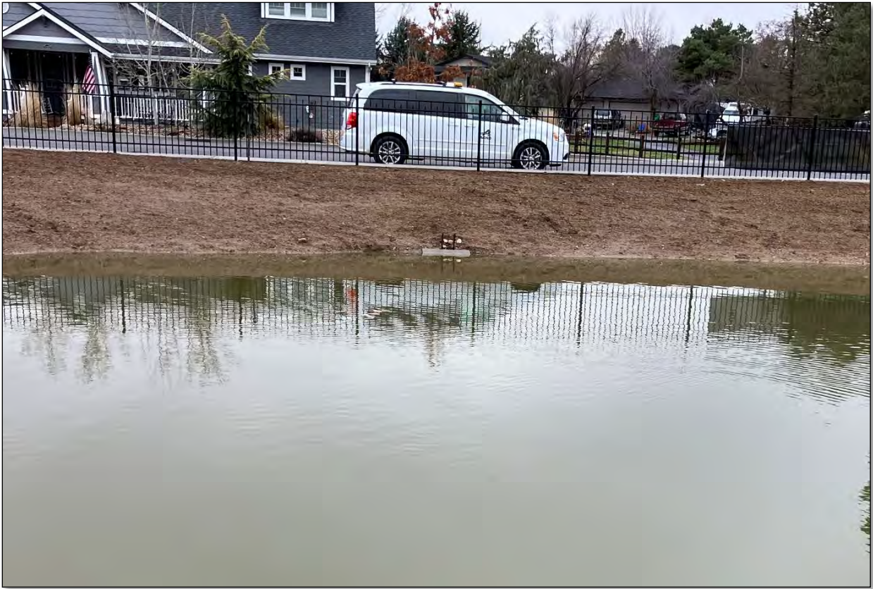
Photo 9: March 2024 – Photo taken facing south showing submerged basin inlet.
