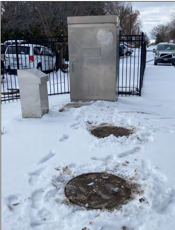
Photo 4 and 5: 11/8/23 - Photos are taken at south end of basin facing west. Photo shows newly installed monitoring station cabinet housing automated sampler and flow meter for stormwater sampling.
