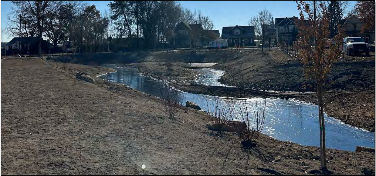
Photo 6: 12/6/2023 – Photo taken facing south showing topsoil, irrigation, and boulders installed. The fence and containerized plants were being installed at the time of the photo.
