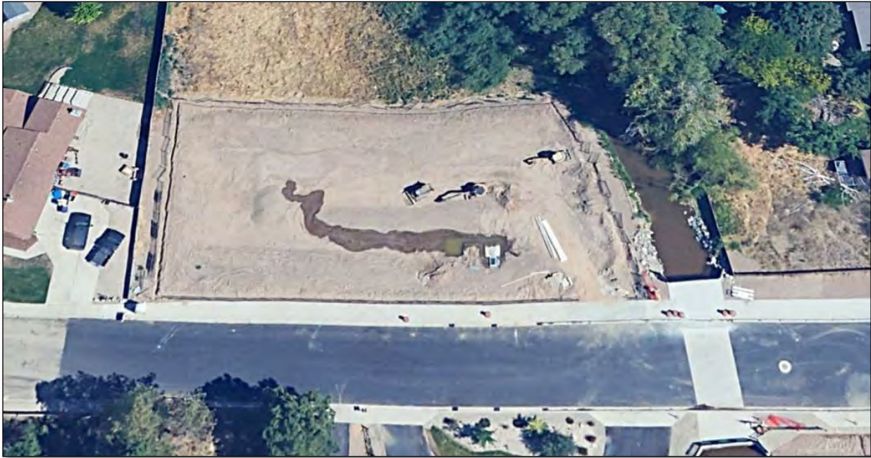
Photo 4: July 2023 – Aerial photo taken facing north showing rough grading and microtopography in progress.
