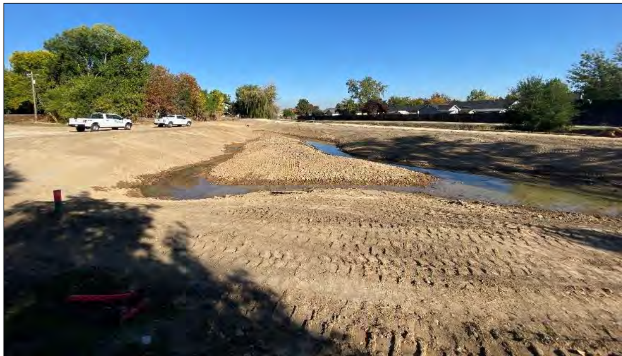
Photo 1: 10/09/2023 - Photo is taken facing north and shows the rough grading and microtopography has been completed.
