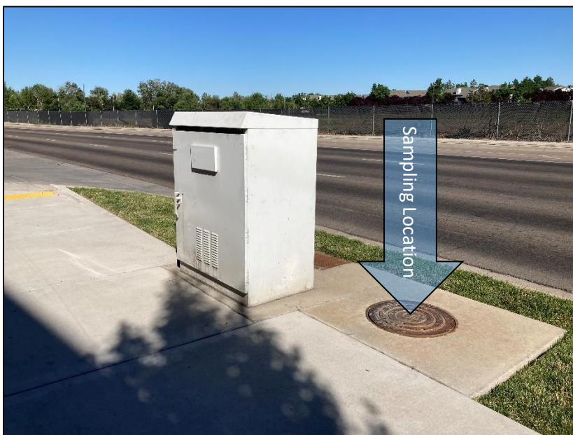
Station setting looking northwest
