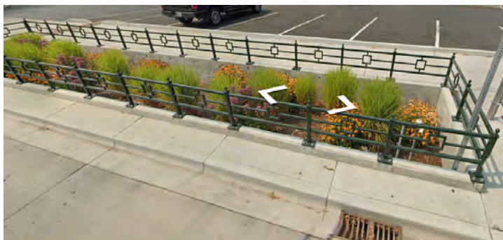
Figure 20: Bioretention Planter at 15th and State in Boise
